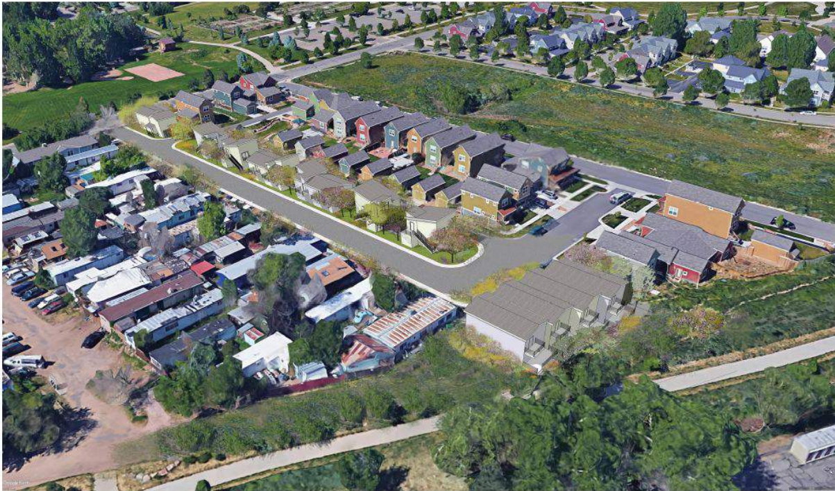
Figure 10 - West End Homes to be built in Phase 1 as per Concept Plan Submittal (August 2018)
