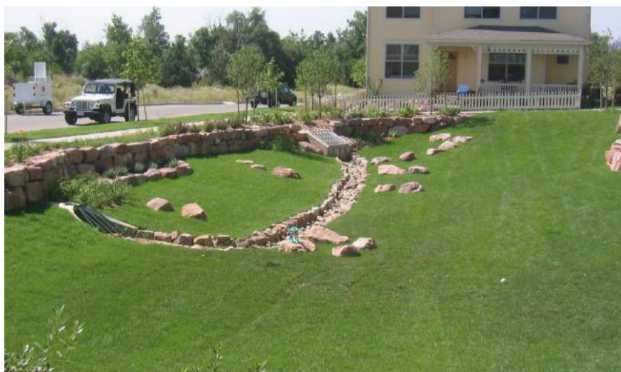
Figure 35 - North Boulder Holiday Development Affordable Housing Alliance Residences Detention/Water Quality Basin
