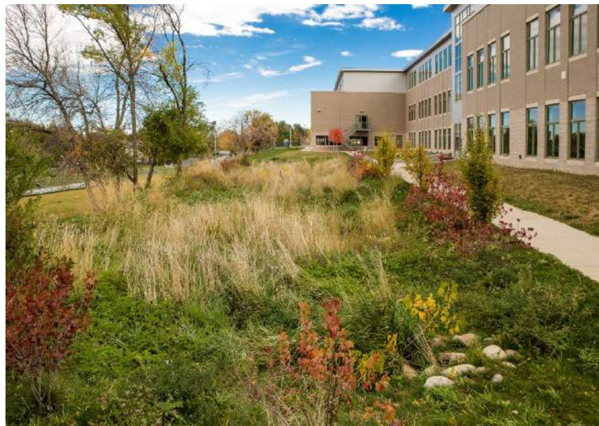
Figure 34 - Casey Middle School Bio-Retention Area
