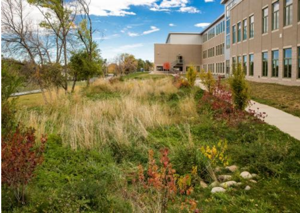
Figure 40 - Casey Middle School Bio-Retention Area
