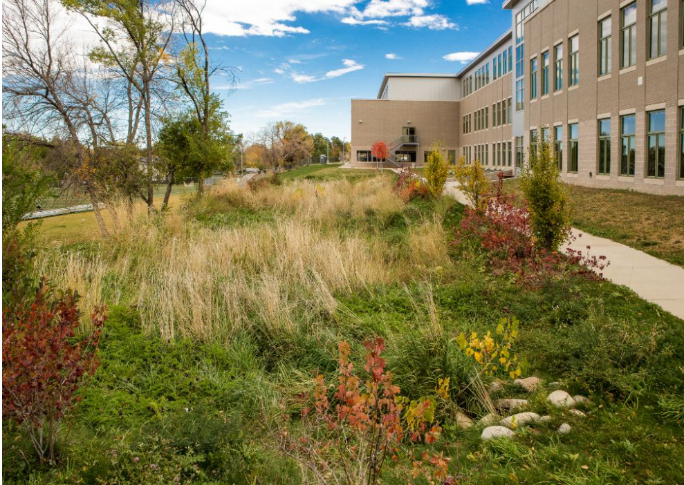
Figure 40 - Casey Middle School Bio-Retention Area
