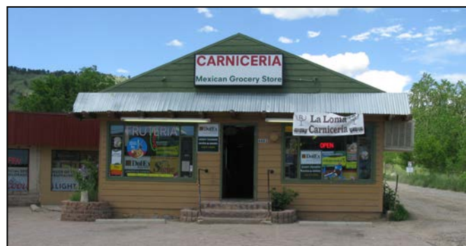
Figure 3: Carniceria Commercial Structure
